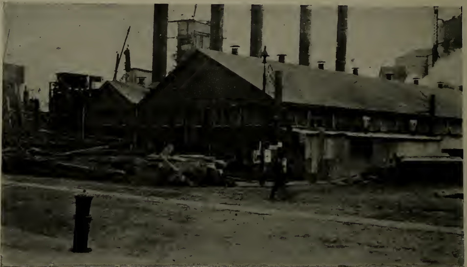
FIG. 4.—Manhattan Power House for P.R.R. East River Tunnels.
